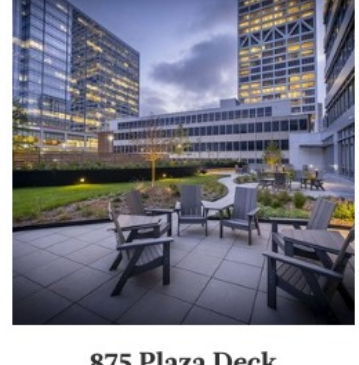
875 Plaza Deck Renovation >
