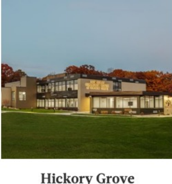
Hickory Grove Community Center >
