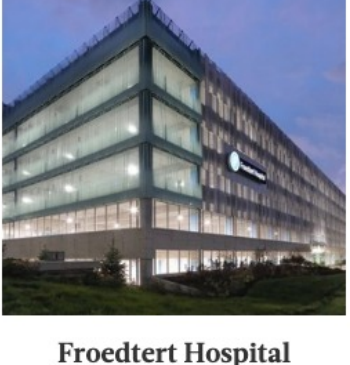
Froedtert Hospital Parking Blue structure >
