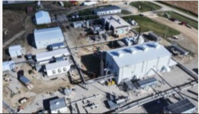
Top Projects of 2025: Wisconsin Reliability Project
